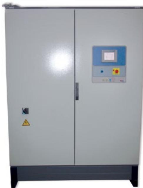
We design and install our control panel according to specific needs of our customers, using any required brand or kind of programming. Our projects respect the legal regulation in force with well-known brands to assure the quality of the project. The touch screen is used for dialogue man-machine (HMI) for an easy change in the modifiable parameters of the installation.
